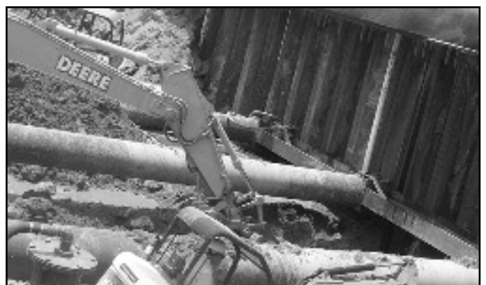
London Avenue Canal breach repair. Photo by John McQuaid, Flickr
