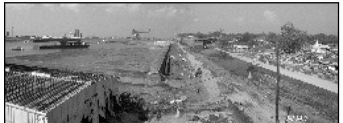
New Orleans 9th Ward Levee damage. Photo by Marvin Nauman, FEMA
