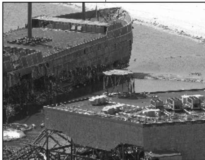
Treasure Bay casino in Gulfport, Mississippi, after Hurricane Katrina struck. Photo by Mark Wolfe, FEMA
